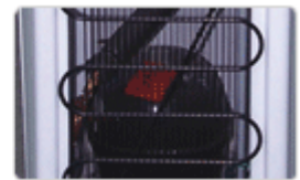
Hermetically sealed reciprocating Compressor
